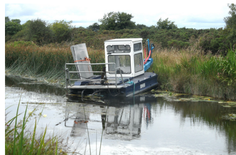
Royal Canal maintenance work near Ballynadrummy.
